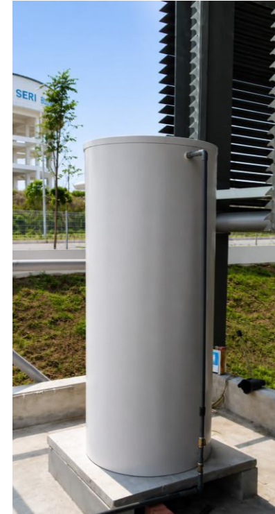
Model in picture (Above) Voda Cylinder 300L 1200mm H, Ø 560mm
